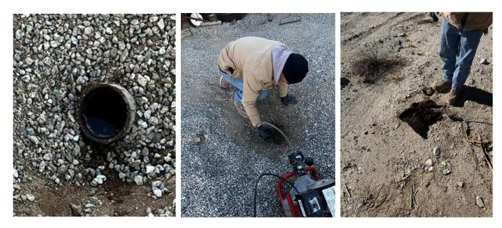
At station #10, the pumps were not pumping, and we decided to rent a trash pump. Due to our trash pumps being used in other stations. Meanwhile someone went to pick up the trash pump at Rent for Rent, sewer jet was used to draft the sewage to prevent a spill.
