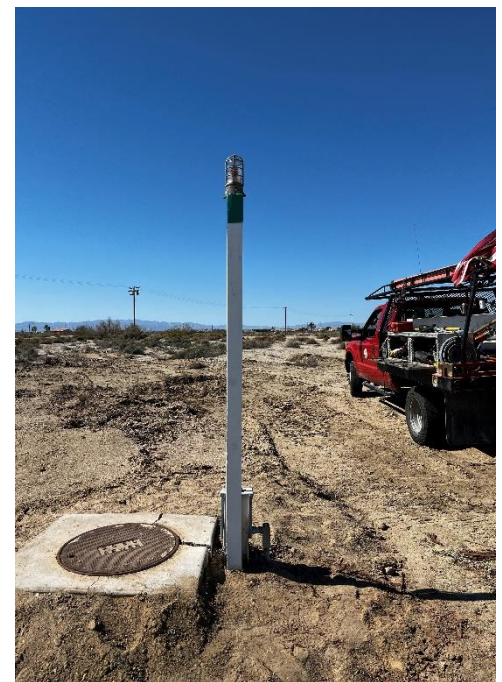
Station #20 a 4x4 pole was installed for the high level light.
