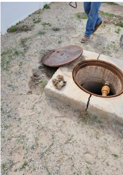
Station #9 high level light on. Residents at Johnson Landing notified employee on call. It was found that the pump was clogged
