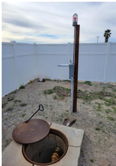
Station #9 high level light on. Residents at Johnson Landing notified employee on call. It was found that the pump was clogged
