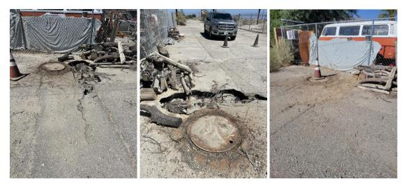
Station #16 force main had a break, crew manage to remove sewer above ground and contaminated soil transported to Lansing facilities. Force main was repaired and was reported to proper agencies.
